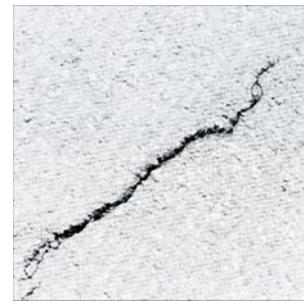
Padding repair of concrete
