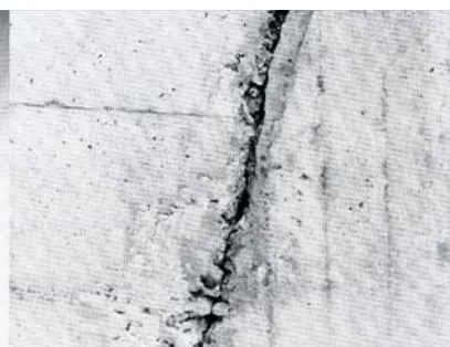
Injection filling to fissure parts of concrete
