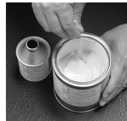
(6) Application of protective coating Add curing agent and stir.
